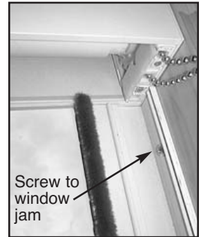
Side channel installed with pocket
